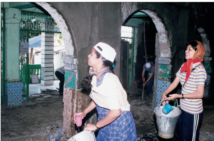
Work in progress at the mosque
